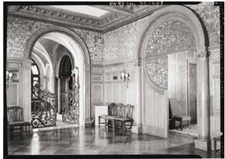
Figure 31. Ballroom, looking toward conservatory and hall (Source: Library of Congress)
