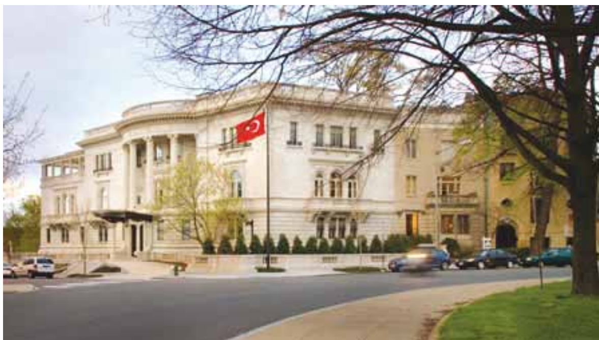
Figure 11. Everett House showing the Sheridan Circle façade (Source: Gary Landsman, fee. Or we can use another photo, just as long as it also shows the Sheridan Circle façade in addition to the main, 23 rd St. facade)
