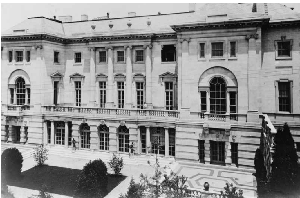
Figure 15. Rear view of Anderson House at 2118 Massachusetts Avenue, NW, showing the Lugarno, a terrace on the mansion's piano nobile (second floor). In good weather, the Andersons used this terrace for outdoor dining and entertaining. The drawing rooms are at the western (left) side of the terrace and the dining room is at the eastern (right) side. Note the high wall and evergreens on the eastern (right) side of the ground-level garden terrace. This wall extends up to the second floor, thereby shielding the terrace from the public view in the alley on that side of the house. Designed by Boston architects Arthur Little and Herbert W.C. Browne in 1901 (construction 1902-1905), the building is now the headquarters of the Society of the Cincinnati. (Library of Congress, Prints & Photographs Division, Historic American Buildings Survey)
